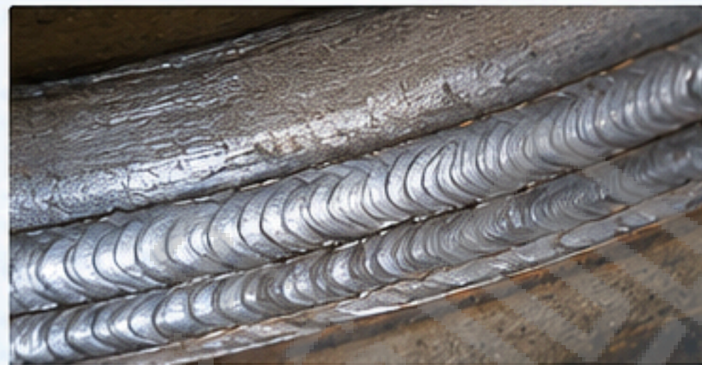
Finished Weld Joint
