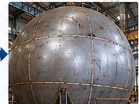
Fit-up and Welding Segment assembly and welding
